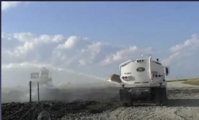
Underground Spill Treatment
