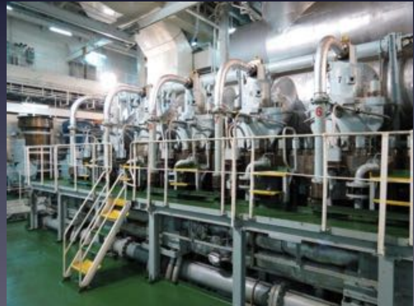
Engine room cleaning
