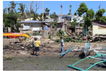
OSEI Associates discussing with Estancia City engineers where start the clean up
