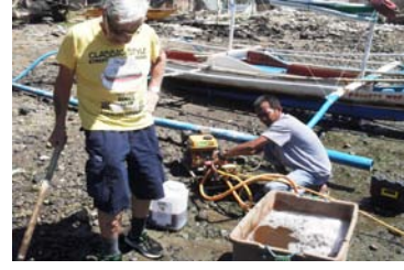
OSE II and water mixed, and the the pumping set up is turned on
