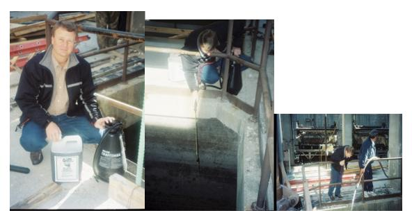
Picture 1 is OSEI Personnel mixing OSE II for application to the RTA wet well or inlet well. Picture 2 is OSEI personnel applying OSE II to the grease floating on the surface of the wet well. Picture 3 is 4 hours after application of OSE II TRA personnel used a water jet to see how well OSE II had caused the grease break up, reduce in size, and to determine if the grease would still adhere to anything as well. The grease had already started breaking up and reducing in size.
