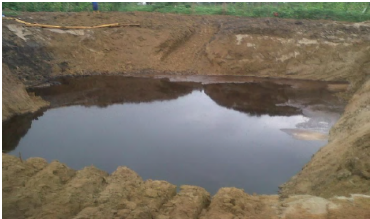
PIT9: EXCAVATED PIT WITH CRUDE BEFORE RECOVERY AND TREATMENT
