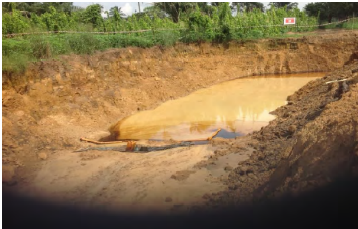
PIT6: EXCAVATED TRENCH OF GROUND WATER CONTAMINATED WITH HYDROCARBON
