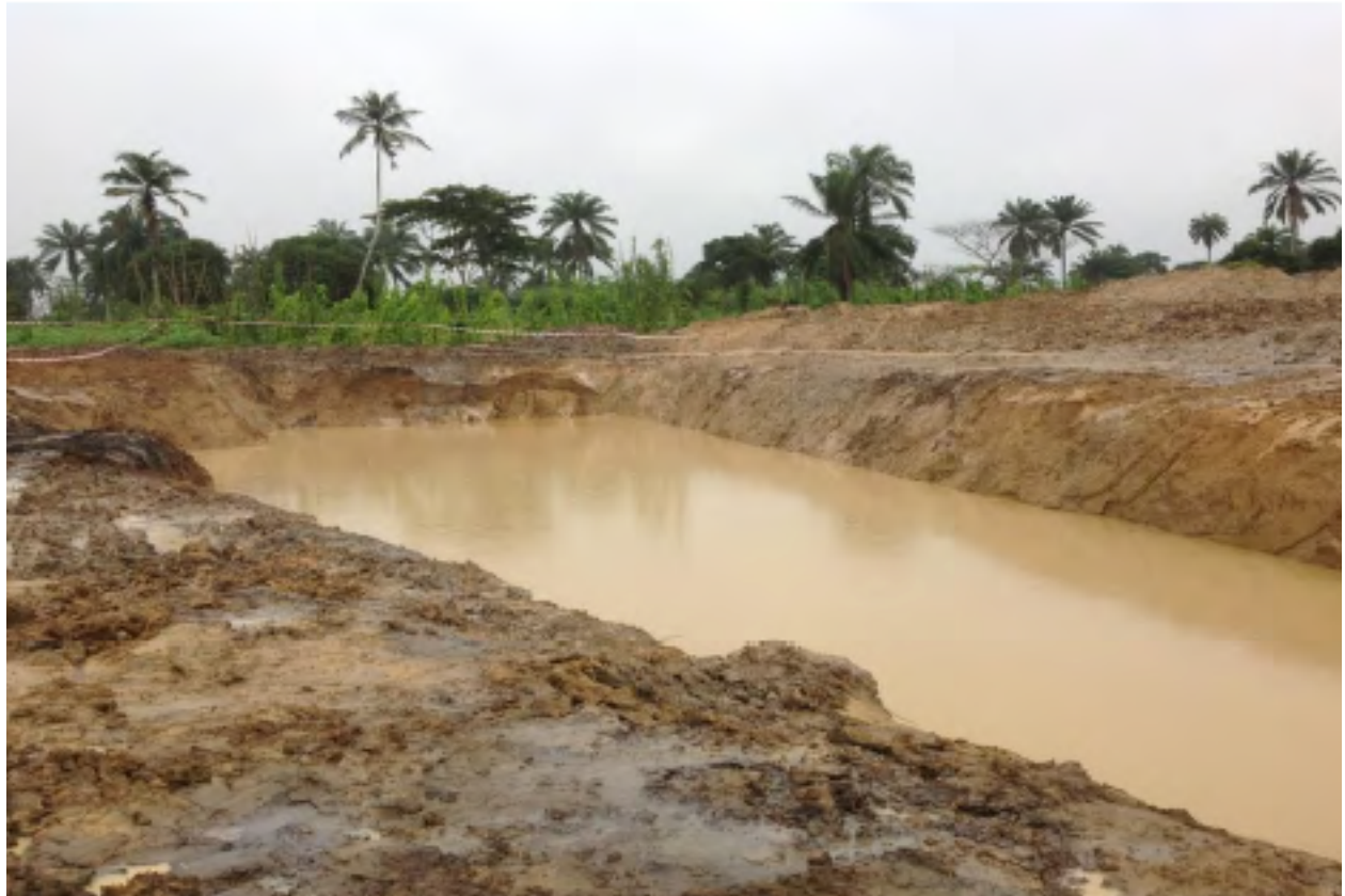
PIT10: AFTER RECOVERY OF CRUDE AND TREATMENT OF EXCAVATED PIT WITH OIL SPILL EATER II
