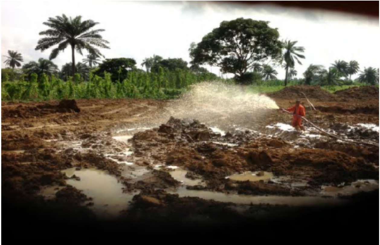
GIOLEE STAFF SPRAYING OIL SPILL EATER II (OSE II) ON CONTAMINATED SOIL
