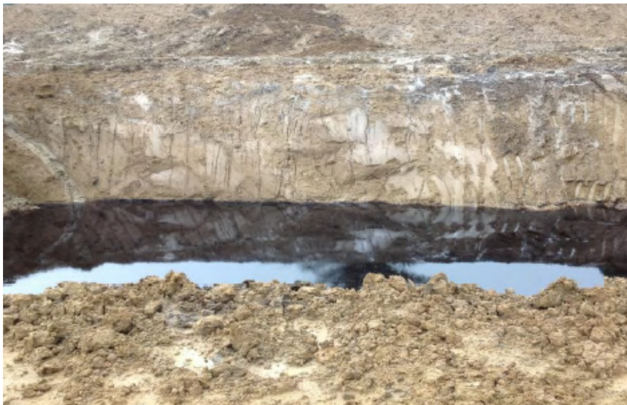
PIT10: EXCAVATED PIT ON SHELL ROW CLOSE TO THE PIPE, BEFORE RECOVERY AND TREATMENT
