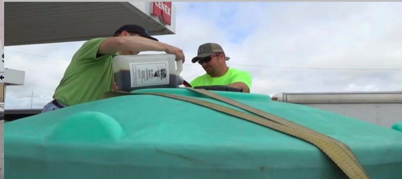
OSE II Added To Aerated Water Prior To Groundwater Injection
