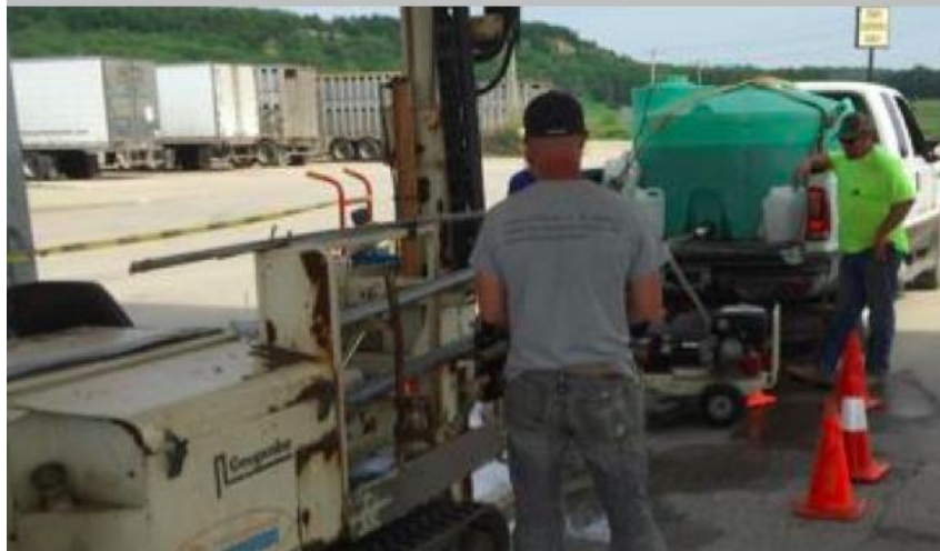
OSE II Injection Process Using The Geoprobe System
