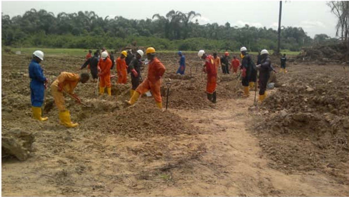
Nigeria, the clean up contractor Giolee Global Resources LTD preparing the soil for application of OSE II
