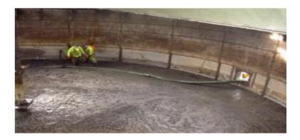
There are two basic means to handle clean up, in a ships fuel Tanks.
