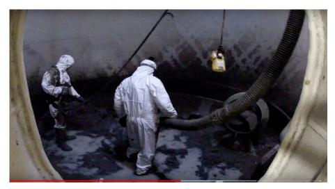
**D.** You will need a circulation pump, with a suction hose and a discharge hose to mix the contaminant in the container to help mix the OSE II and contaminant thoroughly.
