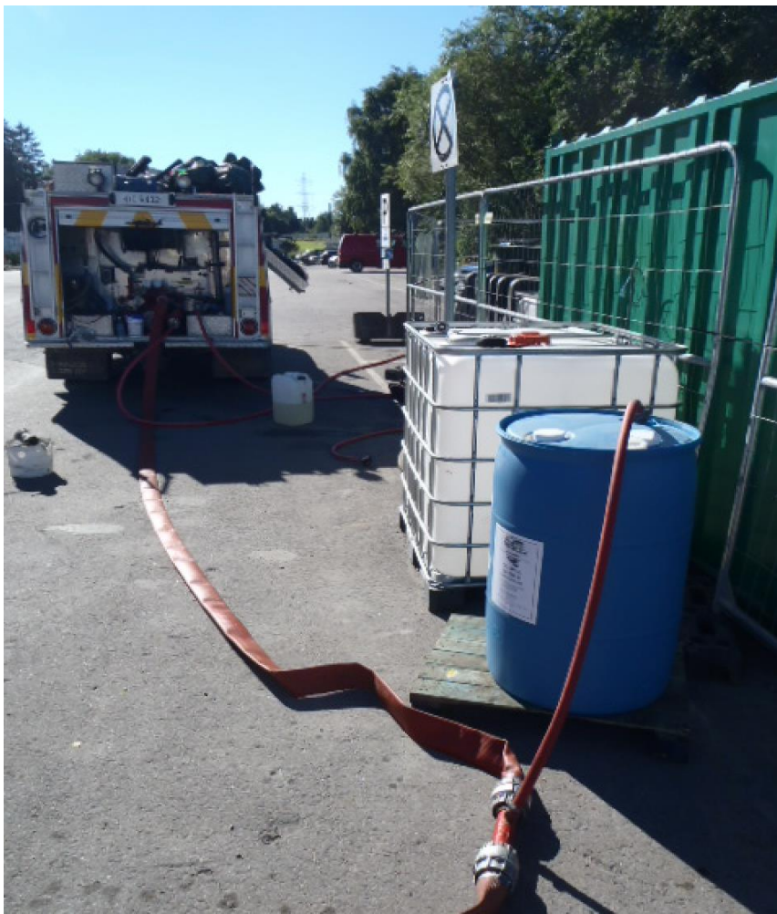
The Fire truck had natural water in its tank, where you can see the water feeder hose, which has another hose pulling OSE II from the Blue drum, where the water and OSE II were mixed at a ratio of 50 to 1, which was injected into the injection holes.
